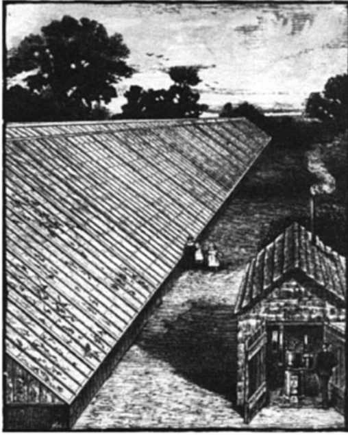
Fig. 2.10 Reproduction from a woodcut dated about 1890 showing the layout of a greenhouse for tomato growing in Guernsey (Channel Islands) with a vertical hot-air pumping engine for the water supply (Source unknown)
